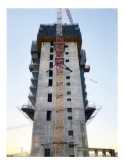
They also used our T-type safety net system, a system for arresting people and objects from falling. This system consists of a safety net attached on brackets for horizontal use.
