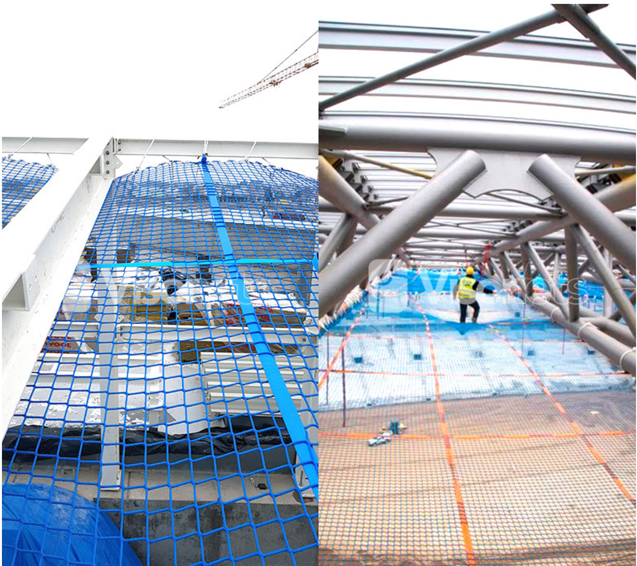
Tensioned Access Platforms (TAP) – Working Platform Nets
